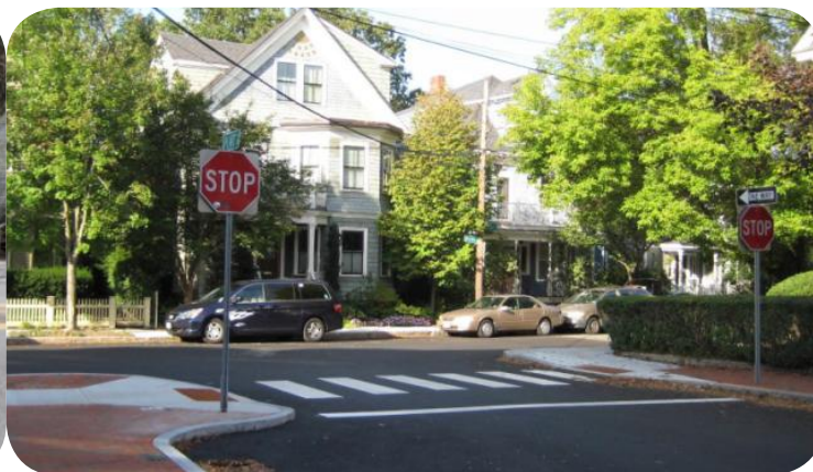
Figure 11. Examples of median refuge (left) and curb extension (right) to shorten crossing distances.
